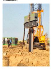
Crane Suspended Vibro hammers: These are more powerful as they get their power from a dedicated powerpack and allow you to drive sheet piles to a depth of even upto 35-40m. This set up is more expensive as you will need a crane with a double winch, a vibro with a powerpack, and a team of crew members for operation of the set up. If you need to drive sheet piles deeper and in hard soils, this is the best set up.
