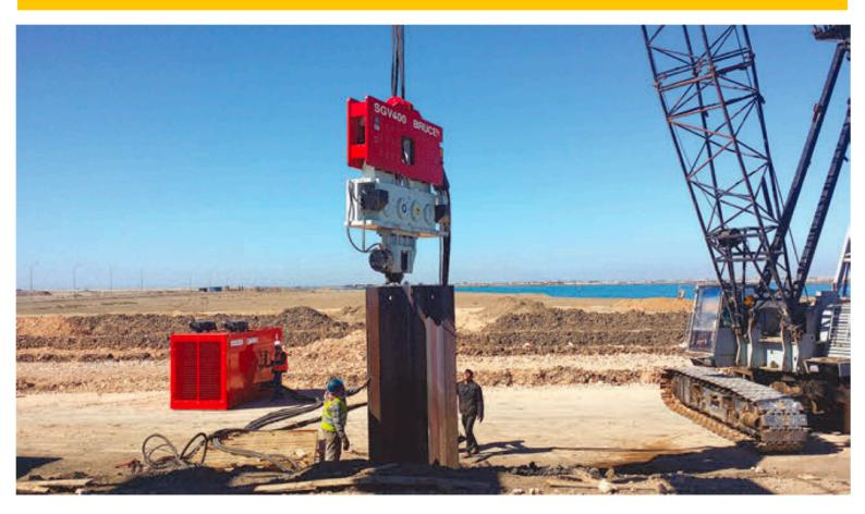
hat is sheet piling? Sheet piles are sections of sheets of Steel or PVC with interlocking edges that are driven into the ground to provide earth retention and excavation support. Vibratory Hammers are usually used to install sheet piles, and Impact Hammers can be used if soils are too hard or dense.
